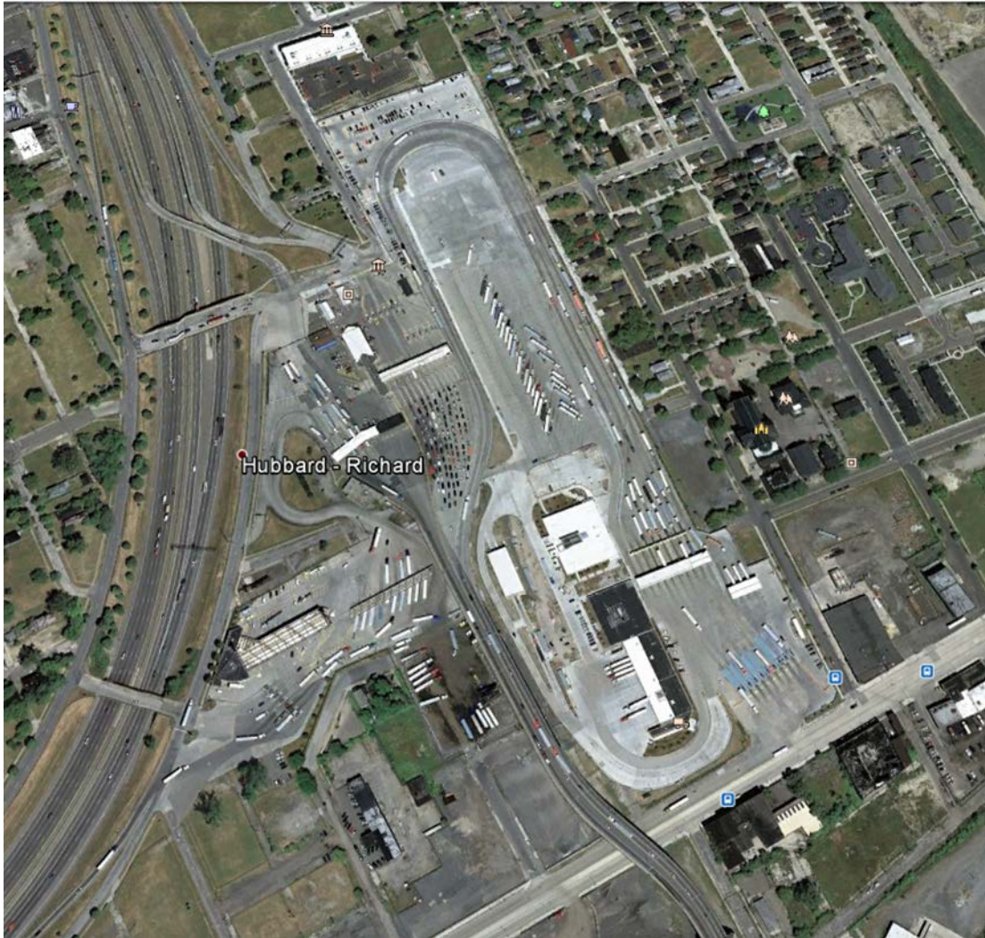
Figure 5-2: The Ambassador Bridge US plazas as of May 2007, before construction began on the Gateway project. Compare the ramp alignment and traffic flow in this aerial image to Figure 5-3 below.
